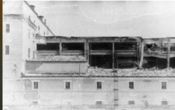
Photo 1. View of Building 201 after the accident.
